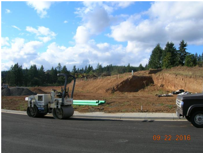
The block of lots facing NW. Note the terraced grading and compare to the more gradual slope shown in the submitted plans.
