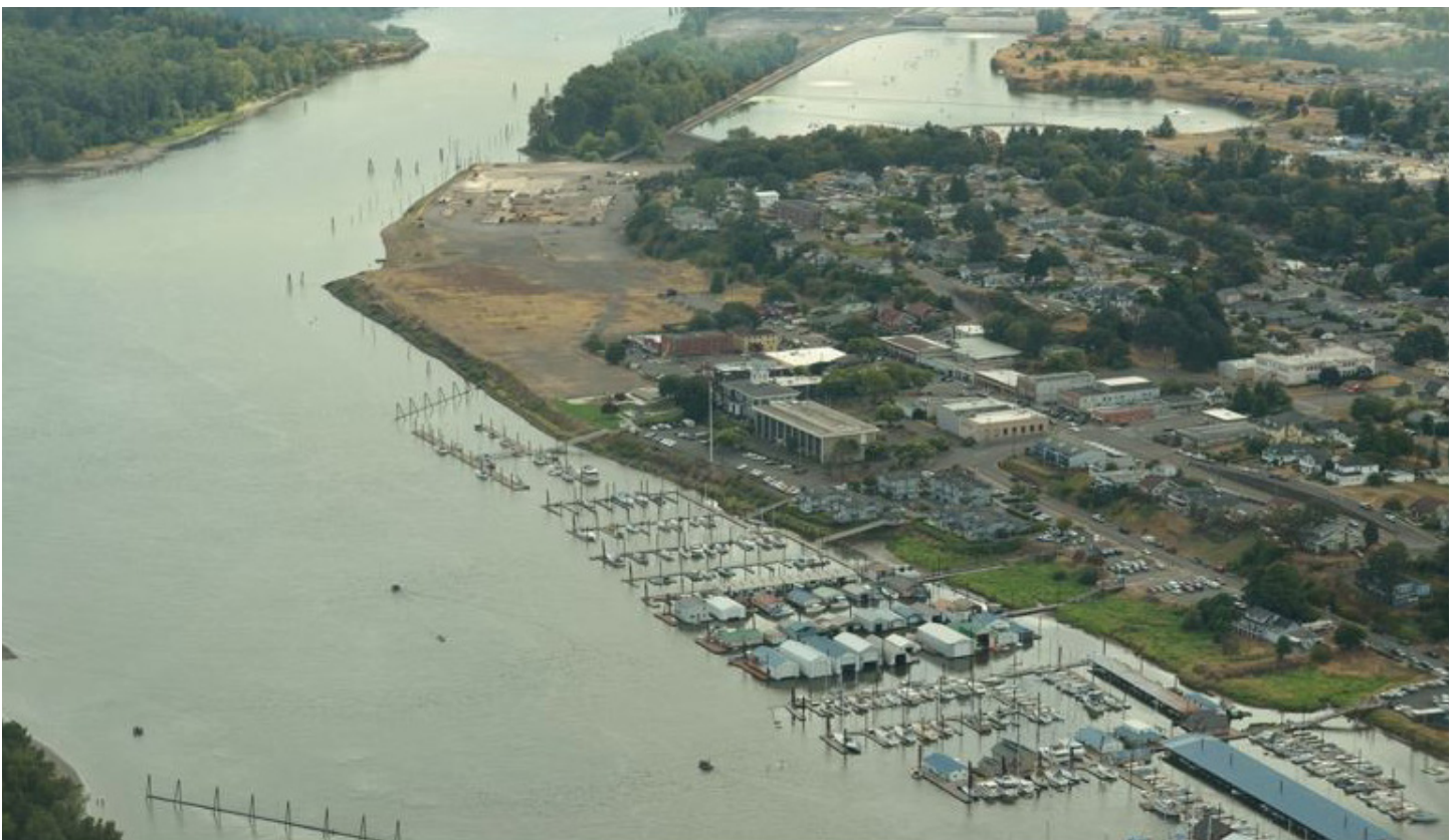
Photograph looking south from downtown St. Helens, across the Veneer Property towards the BWP Property.
