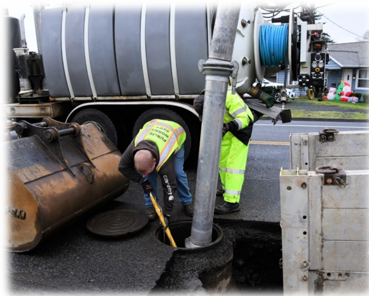
Sewer Main Repair
