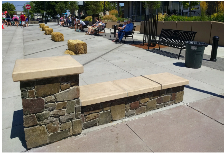
SEATWALL WITH PRECAST CAP
